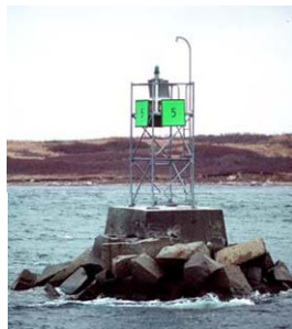
Free Standing Skeleton Tower (Also known as a 1944 tower)
