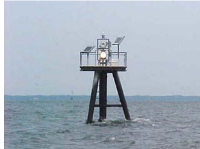
Battered Pile Dolphin
