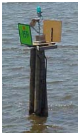
Clustered Pile Dolphin
