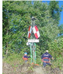
Guyed Skeleton Tower
