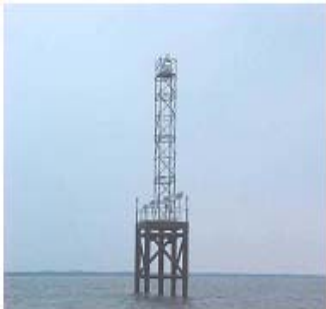
Multiple Pile Platform
